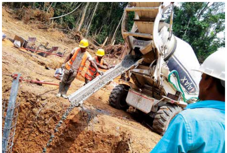
AJAX SLCM working at the construction site
